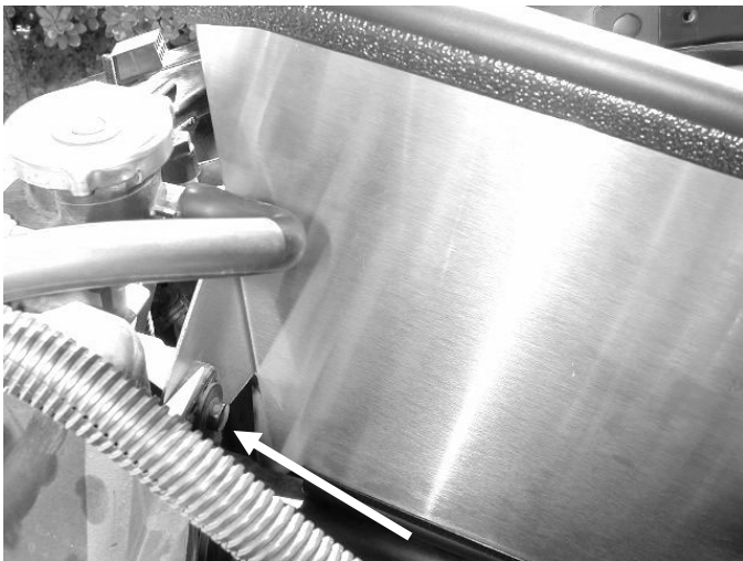
h) Insert the heat shield tab under the radiator shroud tab and secure it with the bolt removed earlier.
